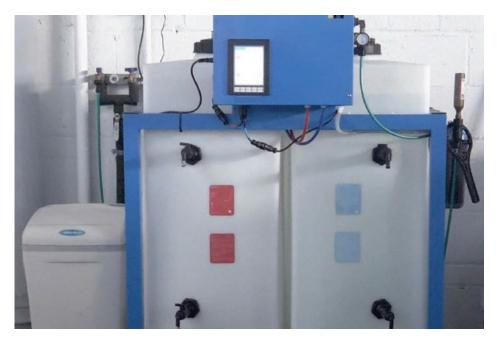
A hypochlorous acid disinfectant and sodium hydroxide generator with a 55-gallon storage tank for each solution in a hospital EVS clean storage room.
